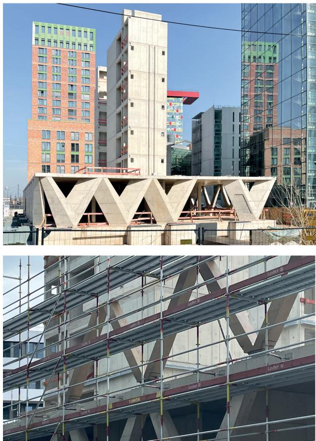
Construction site April 2022: Concreted ground floor and start of timber construction work on upper floors
