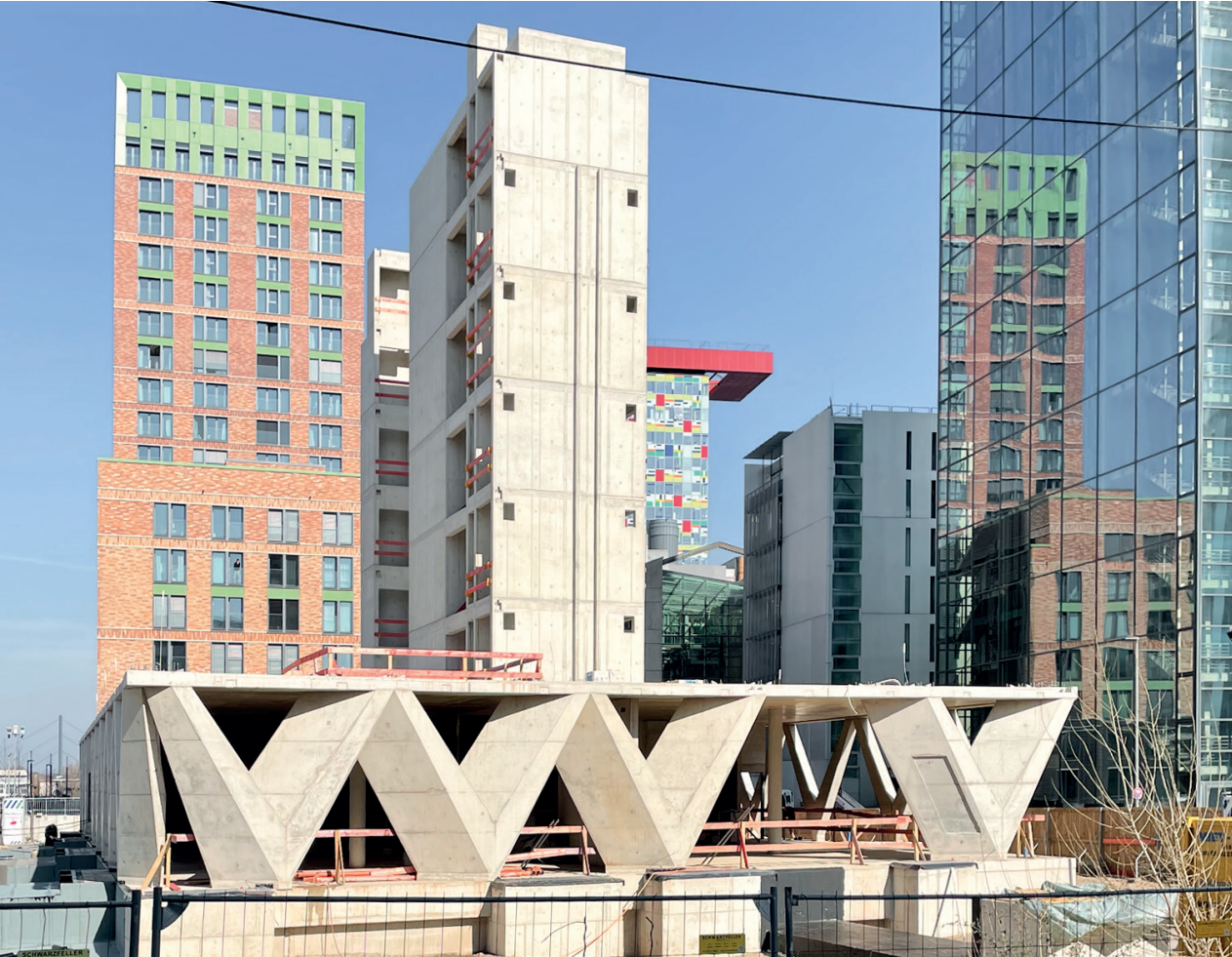
Construction site April 2022: Concreted ground floor and start of timber construction work on upper floors
